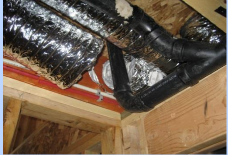
Disconnected Duct
